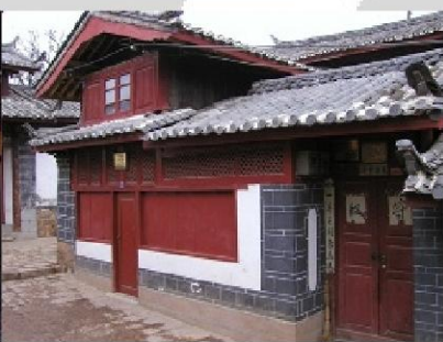
修缮前后照片对比 Photos before and after restoration
